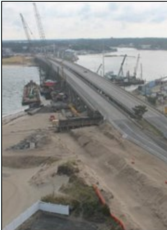
New eastbound bridge lane construction — Jill Doczi
