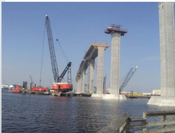
Jordan Bridge replacement.
