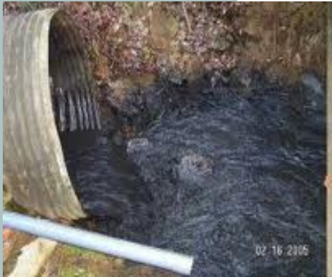
The permanent dredge station will pump sludge from around Virginia Beach waterways to dump trucks in Ocean Park.
